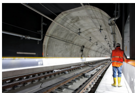
LONE WORKER PROTECTION
